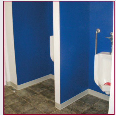
The men's room received new flooring, paint, and countertops. The materials are of a high grade that will stand the test of time.
